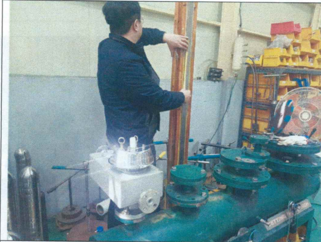
Setting Pressure Check
